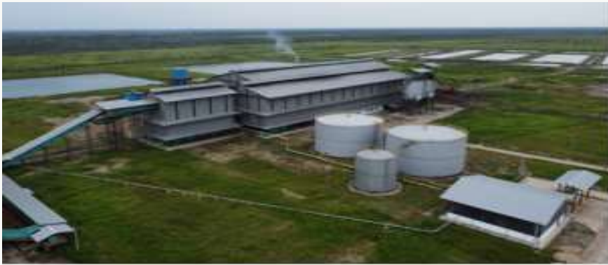
Kaliwang Oil Mill Central Kalimantan, Indonesia
