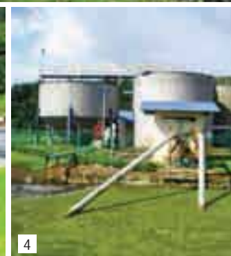
1-2. Good establishment of cover crops on steep slopes and soft ground cover are among the methods to reduce erosion 3-4. The environmental friendly effluent treatment system, which consists of the effluent ponds and bioflow plant, at Genting Indah Oil Mill is capable of treating the final discharge effluent to biological oxygen demand of less than 20 parts per million
