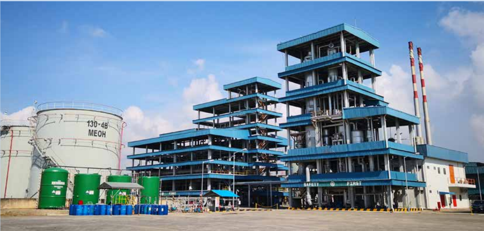
The Group's 2 biodiesel plants – Genting Biodiesel Plant ( top ) and SPC Biodiesel Plant ( bottom )
