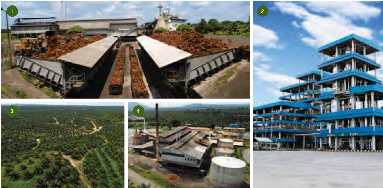
1 & 2. Our Group's oil mills and biodiesel plants are ISCC-certified units. Featured here are (from left to right) Genting Ayer Item Oil Mill, Johor, and biodiesel plant at POIC Lahad Datu, Sabah
