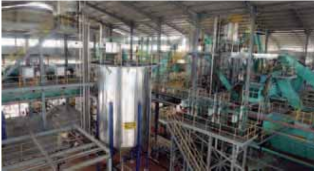
Zero water dilution system to minimise waste generation at Genting Jambongan Oil Mill
