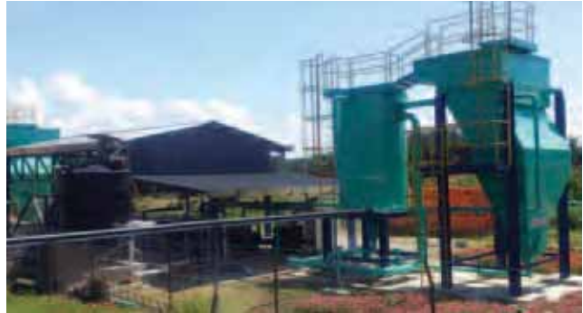
Membrane bioreactor plant treats palm oil mill effluents to ensure biochemical oxygen demand are at permissible levels.
