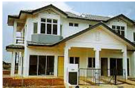
Double-storey terrace houses in Permaipura, Bedong, Kedah
