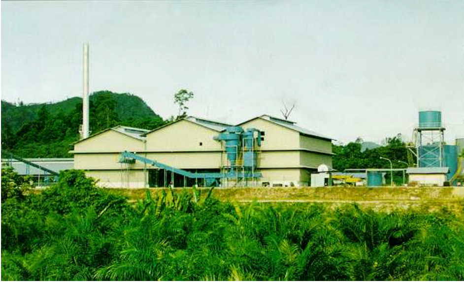
The newly commissioned 30-metric tonne per hour palm oil mill in Serian, Sarawak
