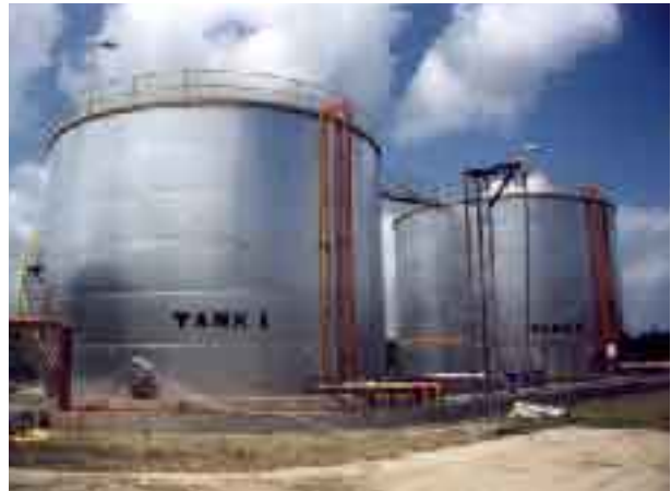
Newly constructed storage tanks at our Sabah mills to cope with increasing production.
