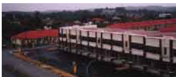
Double-storey shop offices, Indahpura.
