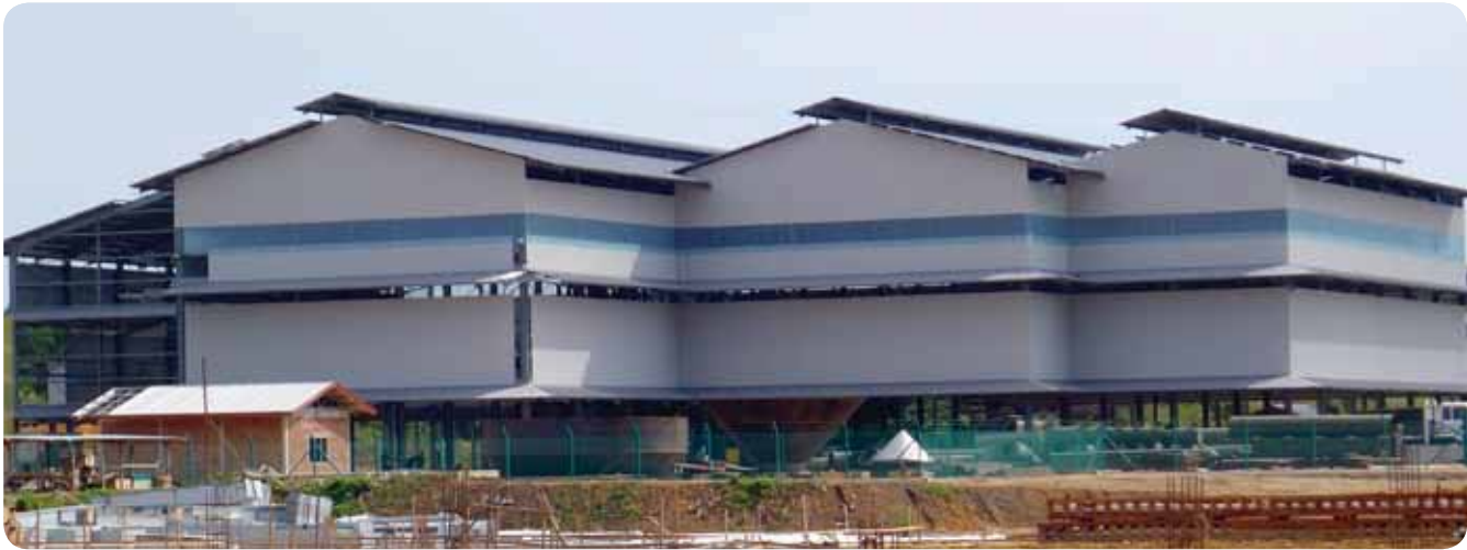
Genting Jambongan Oil Mill – construction of the oil mill is scheduled to be completed by the second half of 2014
