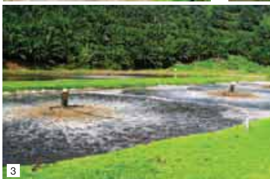
1-2. Good establishment of cover crops on steep slopes and soft ground cover are among the methods to reduce erosion 3-4. The environmental friendly effluent treatment system, which consists of the effluent ponds and bioflow plant, at Genting Indah Oil Mill is capable of treating the final discharge effluent to biological oxygen demand of less than 20 parts per million
