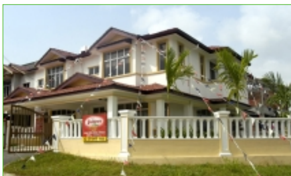
Double-storey terrace houses (Ruby 1), ASIATIC Indahpura
