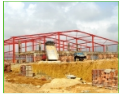
Ongoing construction works at ASIATIC Indahpura Sports Complex
